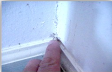
Corners of baseboards
